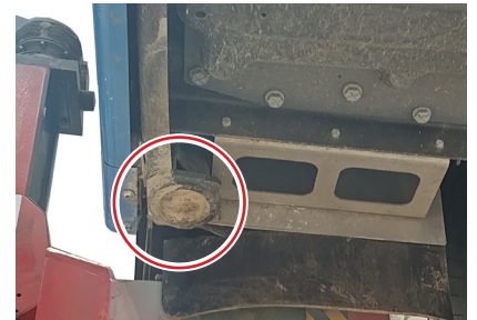
Rear RHS Jacking Point.
