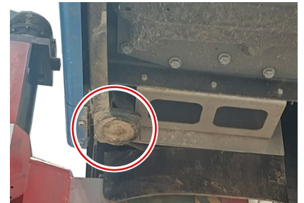
Rear RHS Jacking Point.
