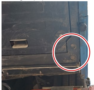
Front RHS Jacking Point
